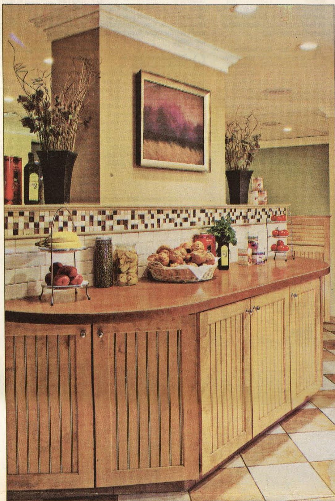
Michael Littlefield fashioned this stained concrete countertop for Popovers Cafe in Portsmouth, N.H., just prior to opening Melange Studio in Kennebunk. The 10-foot-long top to the cafe's coffee station weighed in at about 700 pounds and took 10 people to install.
