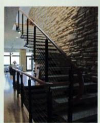
Functional Feature: Sean Dunston, Concrete Jungle Design, Colorado Springs, Colo. — Concrete stairs with decorative texture for slip resistance
